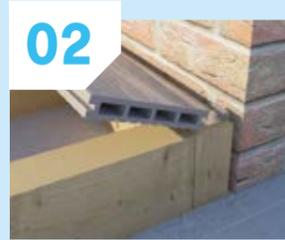
Tilt first deck board so that the leg of the deck locates underneath the lip of the perimeter starter clip.
