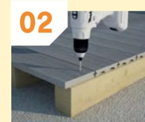
When using the colour matched screws, pre-drill pilot holes first, using a 2mm drill. Ensure pilot holes are no less than 25mm from each edge. Edge boards should overhang the joist by 15mm to cloak the Urban skirting if being used.
