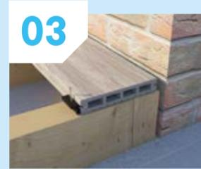
On every joist, position a hidden fixing clip into the groove of the first board and screw into position but do not tighten.
