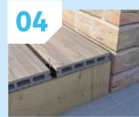
Slide the next deck board into position, locating the hidden fixing clip into its groove. This will set the gap between each deck board. Tighten the hidden fixing clip - but do not over tighten, use a low speed high torque setting on your electric screwdriver.
