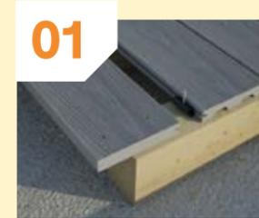
Always use the recommended hidden fixing clips. At the end of the run, an Urban edge board can be used. Fix using a hidden fixing clip and don't over tighten then face fix this board only, using the colour matched screws.
