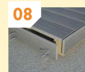
Fix Urban skirt trim underneath the Urban edge board at the joist ends. Leave a 50mm gap between ground and the Urban skirt trim to aid airflow. Use two colour matched screws at every joist.
