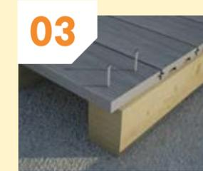
Ensure the colour matched screws are screwed into the pilot holes at 90° with two screws at every joist. Once screwed in place, the head should be flush with the deck surface.
