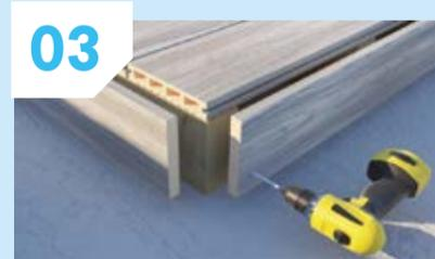
**03** Habitat+ skirt trim can be used to finish the deck on the long end of the boards only. Fix with single screw at 400mm centres. Drill pilot holes before screwing.
